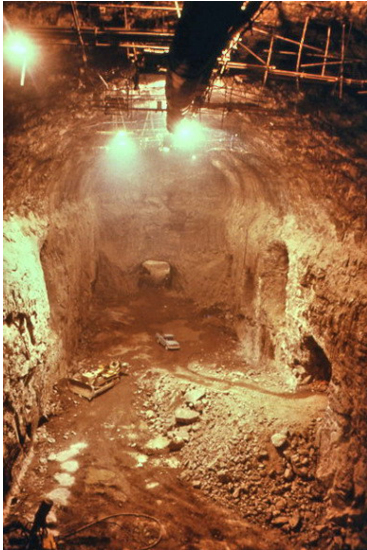
Figure 7: A view of the 25 m span Rio Grande power cavern during excavation of the lower benches.
