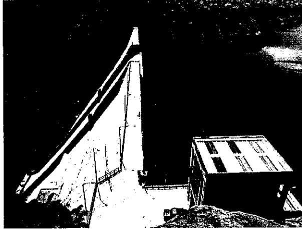
FIGURE 20.5 Miel I Dam in Colombia, which is 620 ft high and used low to medium cement content mixes and no ash. (Photograph courtesy of Ingetec S.A., Colombia.)
