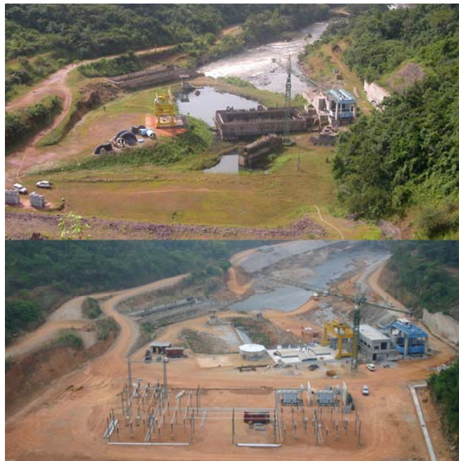
Figure 5-Rehabilitation and completion works in the Powerhouse and Substation area
