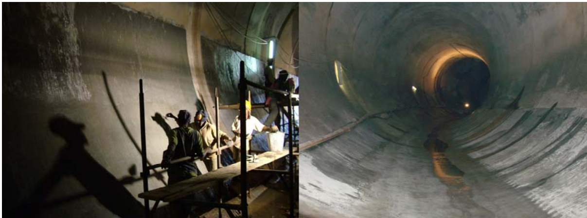
Figure 7-Tunnel rehabilitation works
