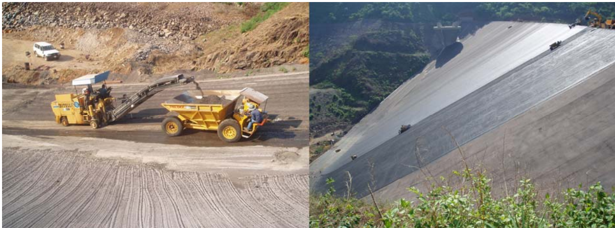
Figure 6–Rehabilitation works of the asphalt concrete facing
