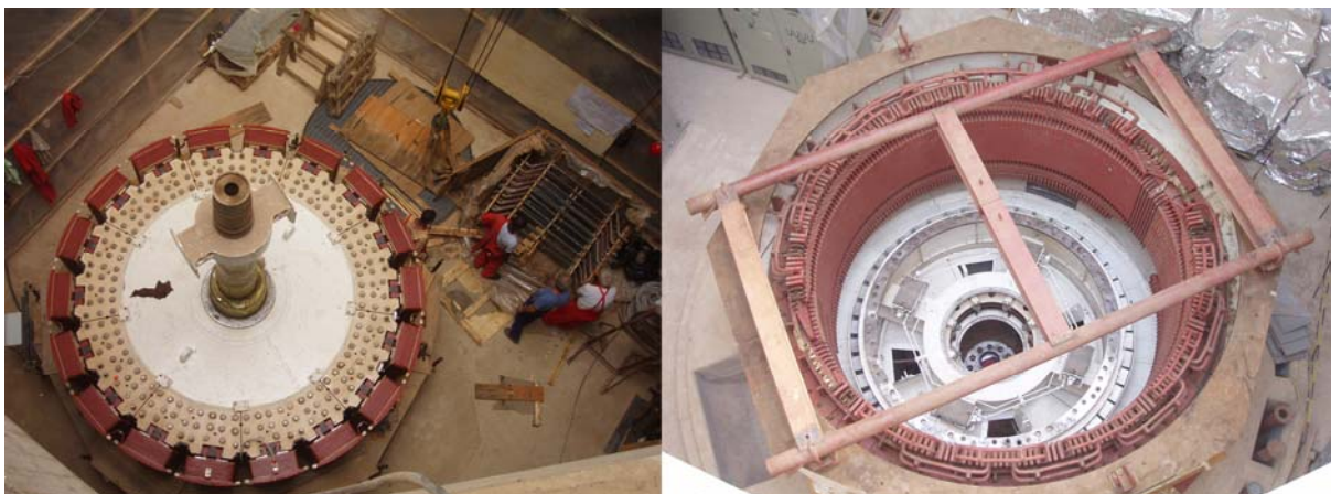
Figure 8-Assembly of generator rotor and stator after rehabilitation
