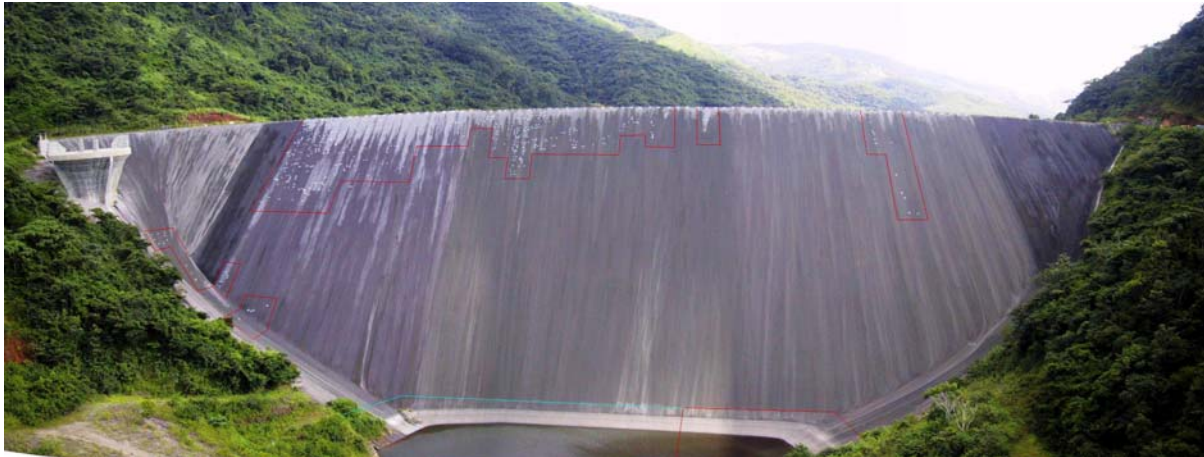
Figure 3-Impervious facing at the end of the interruption period
